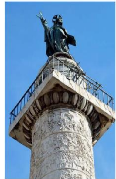
The internal stair case and the viewing platform on the top of the column.
